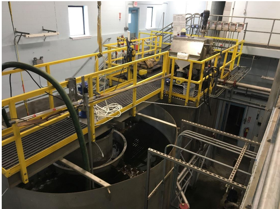
Figure 8: New CoMag® process element (bottom left) located within process building.
