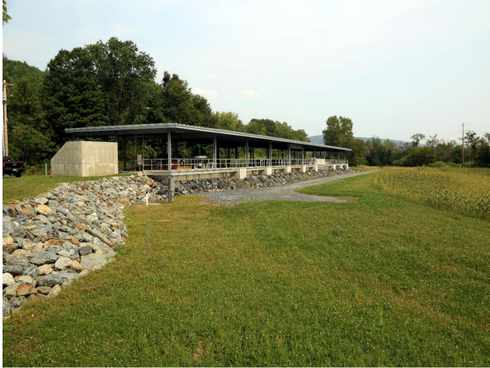
Figure 5: Rear of the new sludge drying bed structure as viewed from the new process building.
