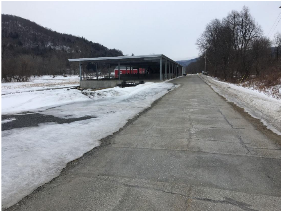
Figure 4: New covered sludge drying bed structure (with new process building in background).
