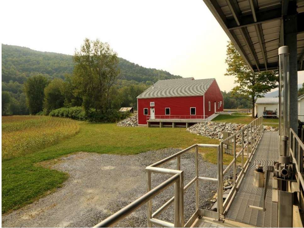
Figure 3: New process building as viewed from the rear of the new sludge drying bed structure.
