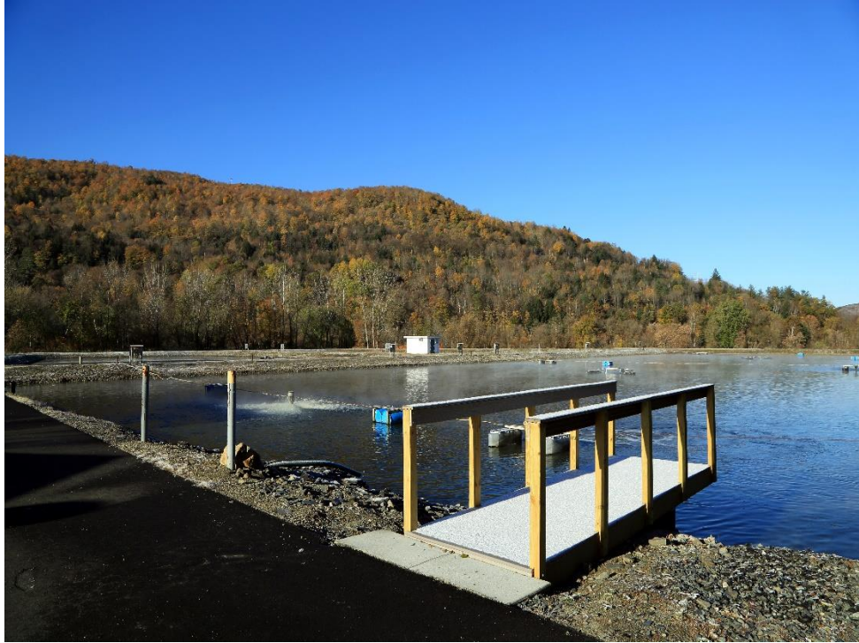
Figure 1: Existing aerated lagoon system.
