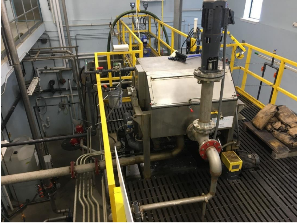
Figure 9: Magnetic drum separator (removes magnetite from CoMag® treated wastewater).
