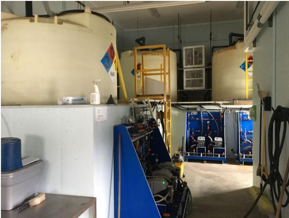
Figure 10: Chemical (PAC, \text{FeCl}_3 & \text{NaOH} ) storage tanks utilized during TP removal process.
